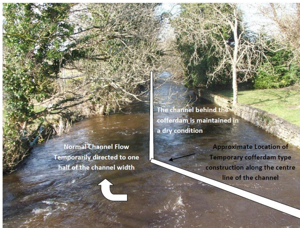
Figure 4.4 - Proposed Works Channel Works in the vicinity of Craughwell Village and sketch of cofferdam location
